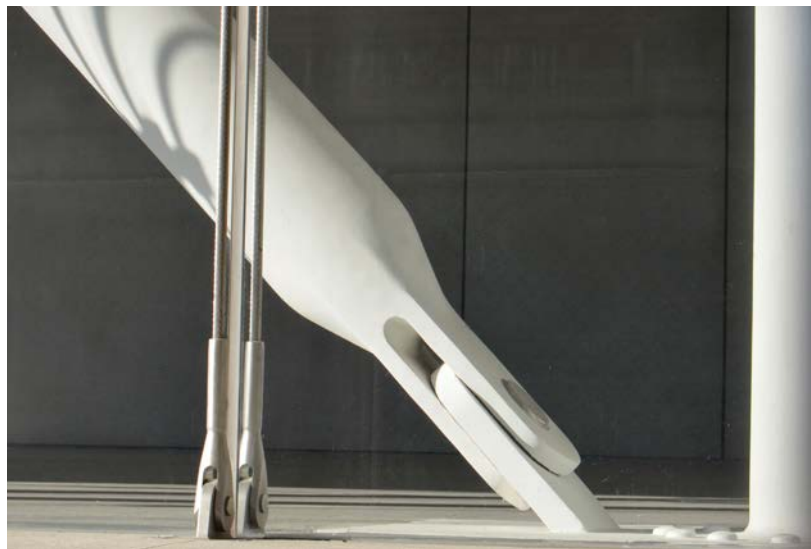
Figure 1.5 CAST CONNEX® Universal Pin Connector™ at a CHS brace member end with cast stainless steel cable fork ends in the foreground in the Whitney Museum in New York, NY
