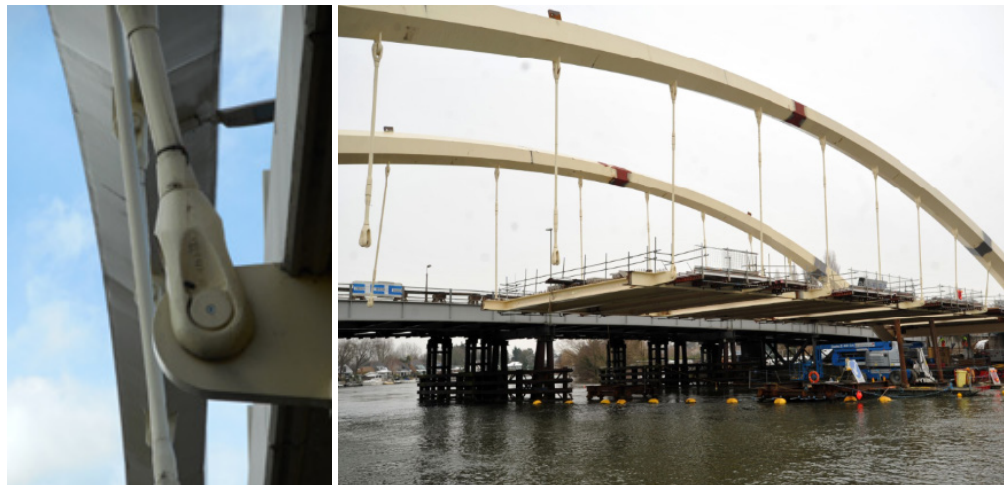
Figure A.17 Detail of tie rod connection and construction sequence
