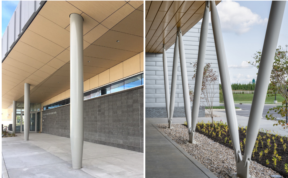
Figure 1.6 CAST CONNEX® Architectural Taper™ at a CHS column end (left); CAST CONNEX® Universal Pin Connector™ + Architectural Taper™ at CHS member ends (right)
