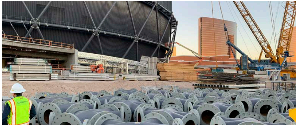
Figure A.5 Cast nodes on site ready to be installed
