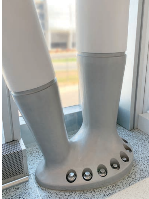
Figure A.13 Cast steel base in-situ
