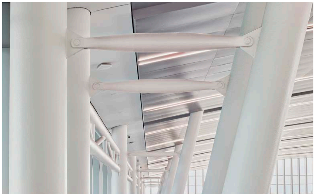
Figure A.14 Standardised cast steel Architectural Taper and Universal Pin Connectors by CAST CONNEX were used to connect the lateral bracing in the long span roof at the top of the columns and in bracing orthogonal to the frames
