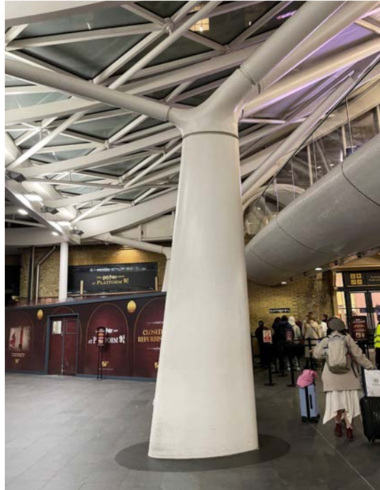
Figure A.3 Cast nodes connect the 'branches' to the 'trunk' columns
